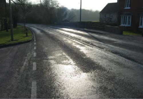
Highly polished surfaces often mean low skid resistance
